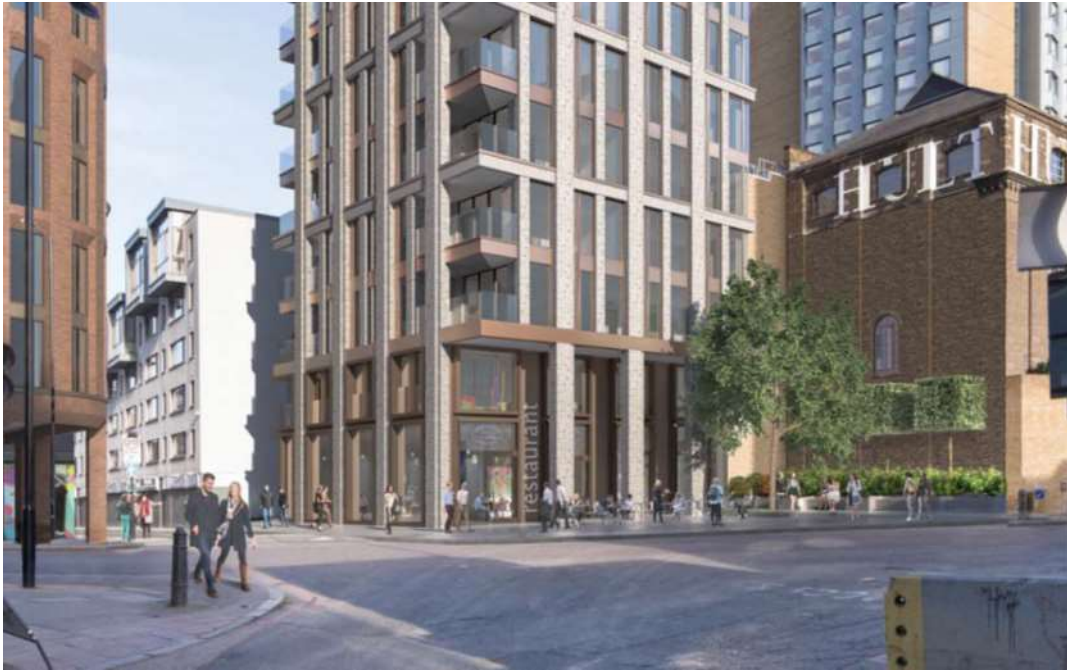
Figure 5: Image of scheme from Alie Street with the exposed foot of the listed brewery building (in right of image)
