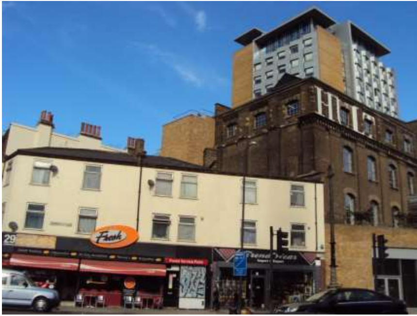
Figure 2: No. 29-31 Commercial Road (with listed former St George's Brewery Road right hand side of photo and the student block at No. 35 Commercial Road set behind warehouse)
